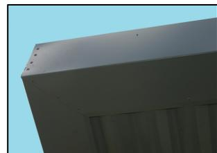
For the capping along the run of the roof, rivet at 300mm centres, aligning with the stitching screws. Silicone the corner capping joins top, side, and bottom to ensure no leaking. Use only neutral cure silicon. All holes for rivets will need to be pre-drilled.
